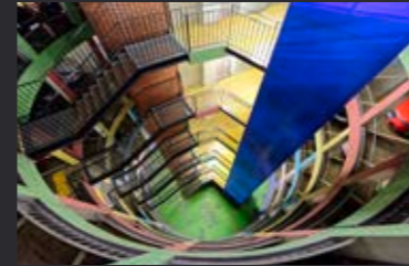
Parking de Rive
